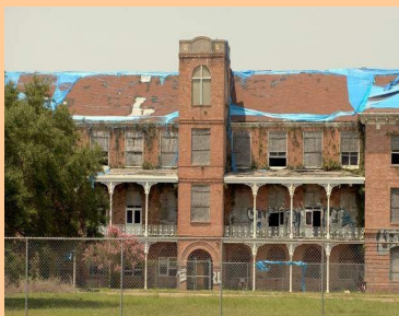
3. Holy Cross Administration Building
